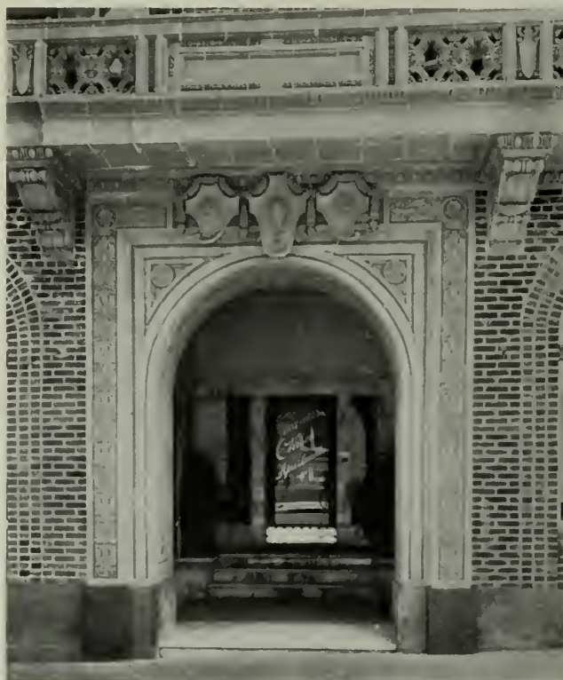
DETAIL OF ENTRANCE, CHISMORE APARTMENTS.
